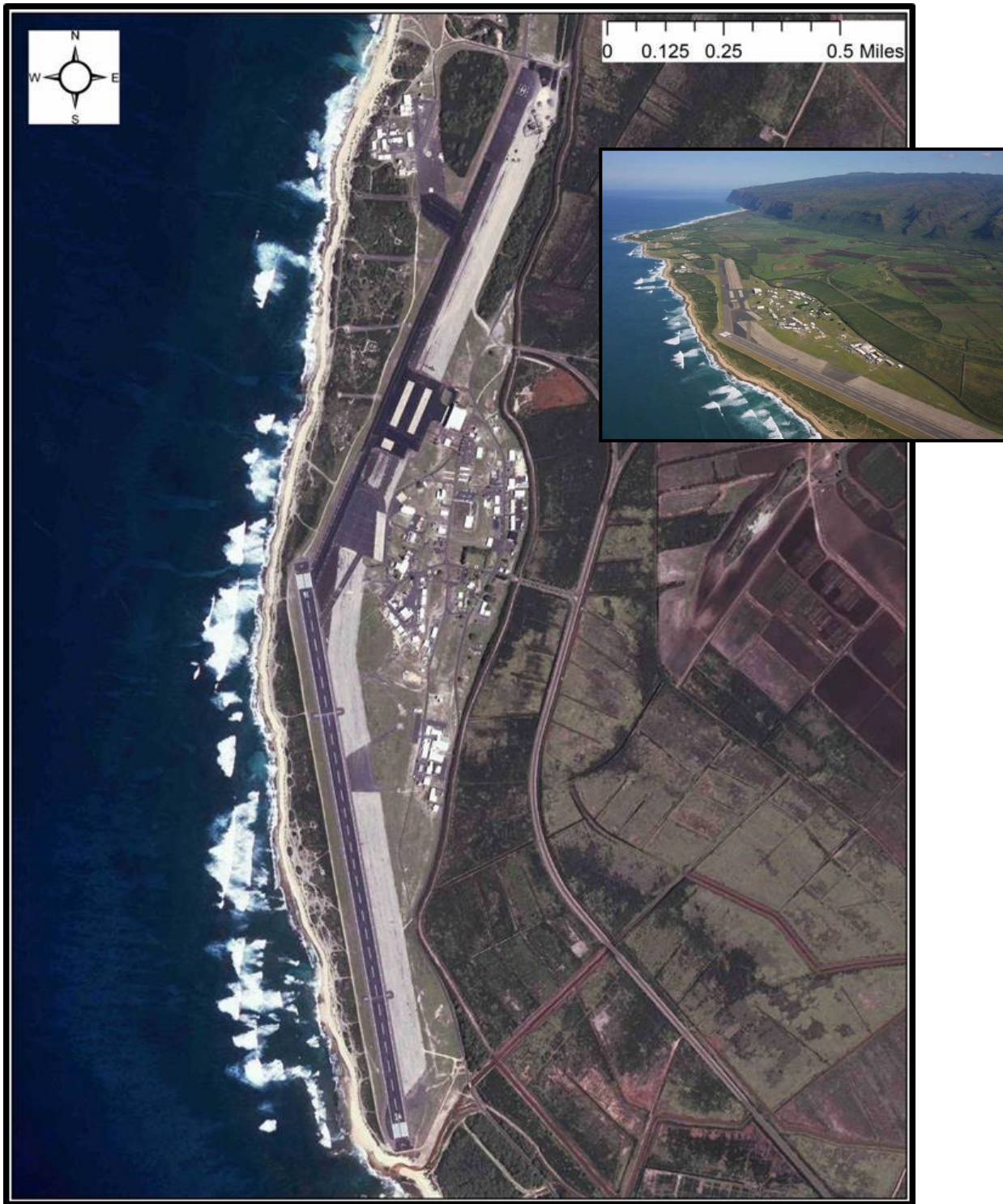
Figure 2. Aerial views of airfield area of PMRF with Kini Kini and Kawaiole Ditches (bottom) and agricultural lands visible (right)
